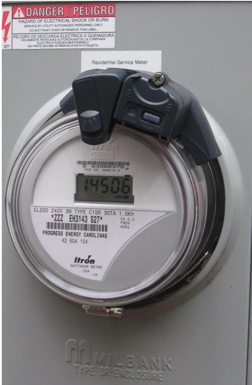
Figure 7 – Blueline PowerCost Installation
