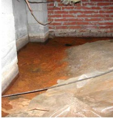
**FIGURE 16** Significant amount of water pooling along perimeter of crawl space wall
