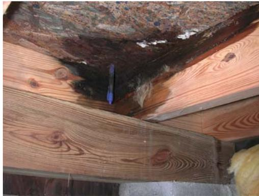
**FIGURE 32** The rot illustrated in this picture could have resulted from a condensation event
