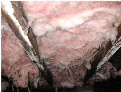
**FIGURE 39** Fallen insulation reveals a floor penetration.
