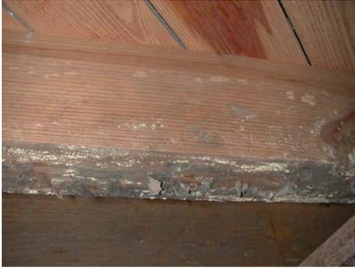
**FIGURE 30** The wood moisture meter reading of 20.6 is at mold-forming levels and could explain the growth on the wood framing
