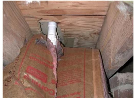
**FIGURE 40** Fallen insulation found on crawl space floor.
