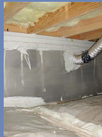
closed R19 floor insulation
