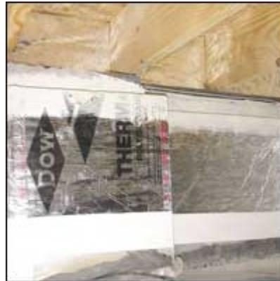
This wall-insulated closed crawl space uses 2-inch thick foam insulation (R-13), with the termite inspection gap left uninsulated.
