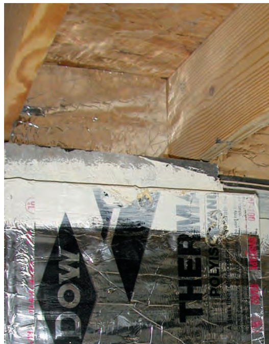
This wall-insulated crawl space uses 2-inch-thick foil-faced polyisocyanurate insulation. The foam plugs in the band could be replaced by sections of batt insulation. A termite inspection gap is visible at the top of the wall insulation.
