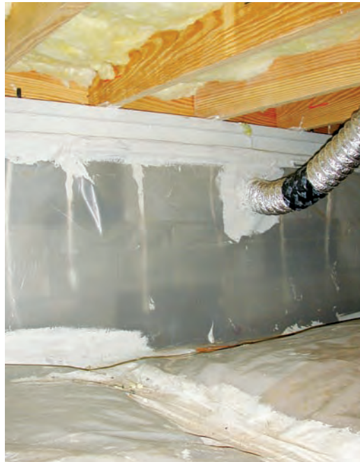
This floor-insulated crawl space has a termite inspection gap at the top of the vapor retarder. Note that penetrations are thoroughly sealed with mastic.
