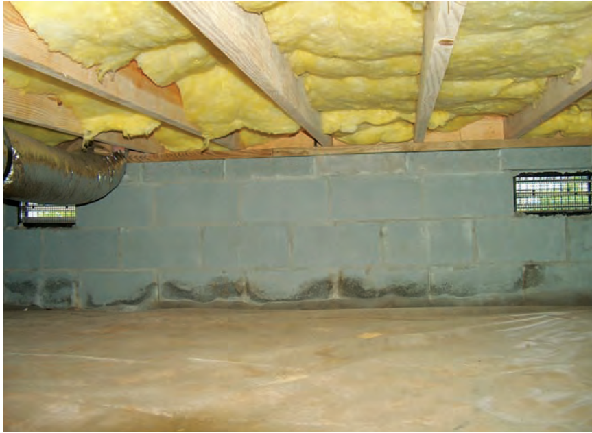
The wall-vented control houses in this study have much better crawl spaces than the typical crawl space we encounter in the field. The control houses have well-installed insulation and 100% ground vapor retarder coverage of the soil, and no problems with intrusion of liquid water from outside.
