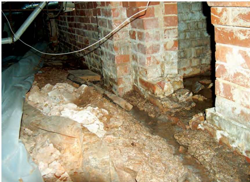
A more typical vented crawl space in North Carolina exhibits water leakage, poor drainage, a low-quality vapor retarder, if any, and various complications such as attached under-porch areas.
